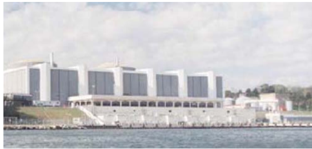
Maryland has worked hard to build partnerships that promote the resiliency of privately-held infrastructure such as the Calvert Cliffs Nuclear Power Plant.
